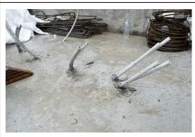
Manual labour required to finish around closely spaced tubes. Tube numbers multiply quickly, depending on starter bars specified by the head consultant.
