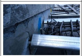
The wall end usually requires some cutting to allow the addition of a grout tube.
