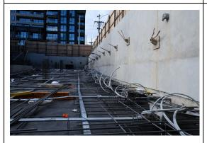
Every sleeve and tube requires two individual grout tubes. This creates havoc when finishing the slab, as concrete finishers need to work around all of the tubes, delaying the process.
