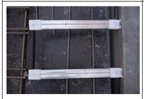
Two sleeves connected in series allow grouting to enter at sleeve one (wall side), and exit at sleeve two (wall side). Reducing the number of grout tubes and locating them at the slab edge, facilitates quick trowel finish of the concrete slab.
