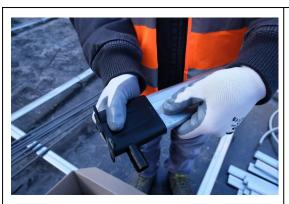
SleeveCap installed on a typical Post Tensioning duct; snug fit, prevents concrete from entering.
