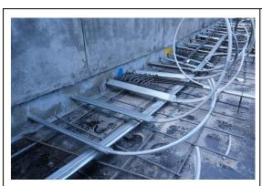
PT Duct cut to length and grout tube duct taped to the end, to allow grouting later.
